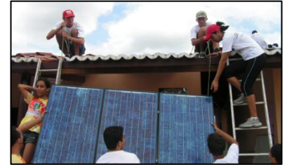
A USAID-supported program trains youth in Brazil to install solar panels.
